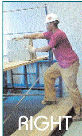
Step to it – When moving heavy materials manually, an elevated platform can help prevent stress and strains from unnecessary bending and twisting.
