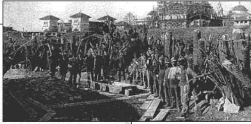
Laborers lay a waterline for the Exposition.
