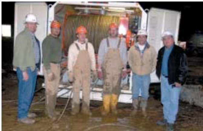
Building a new casino in Salamanca are, from left, Donald R. Giardini, Local 621 business manager; John White, Jake Hill and Jim Phearsdorf of Local 621, Jon Lichy, vice president of Sue-Perior Concrete and Paving Inc., and Steve Gordon, SNI TERO compliance officer.
